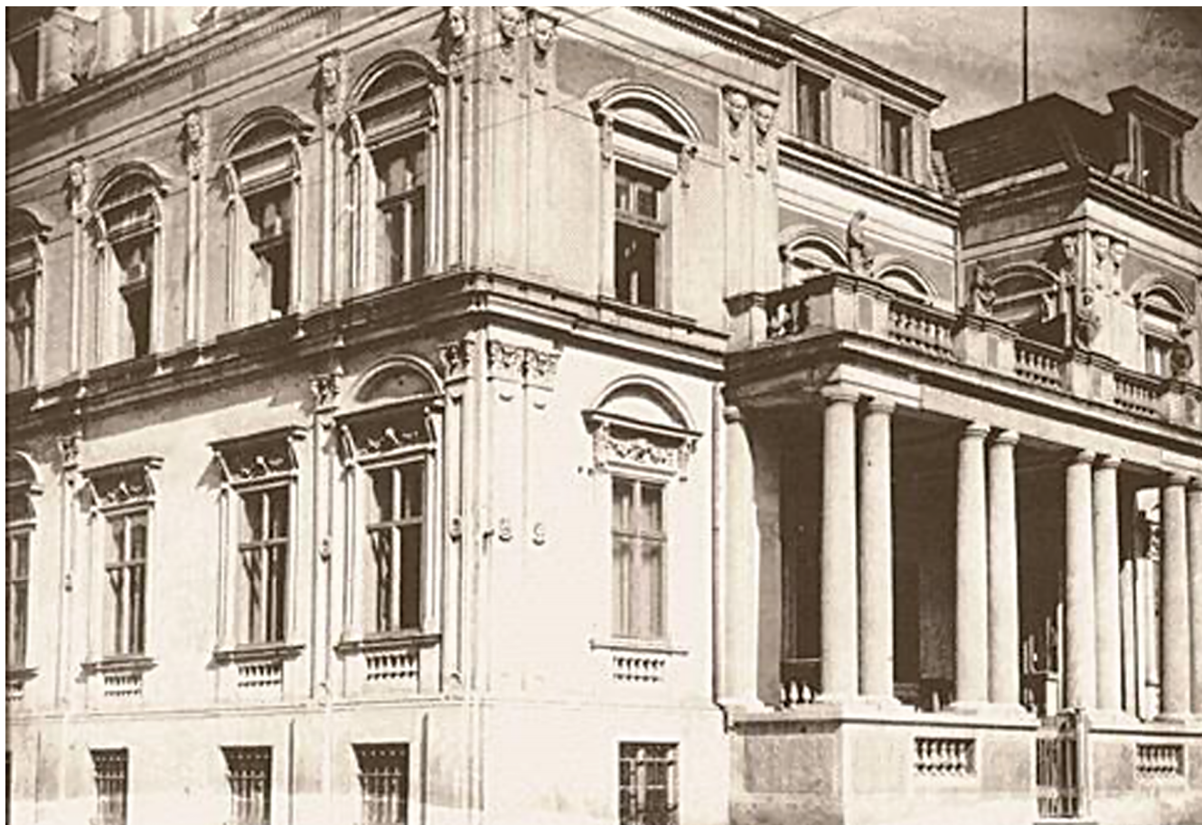
Building of the National Library at Kosancicev venac
