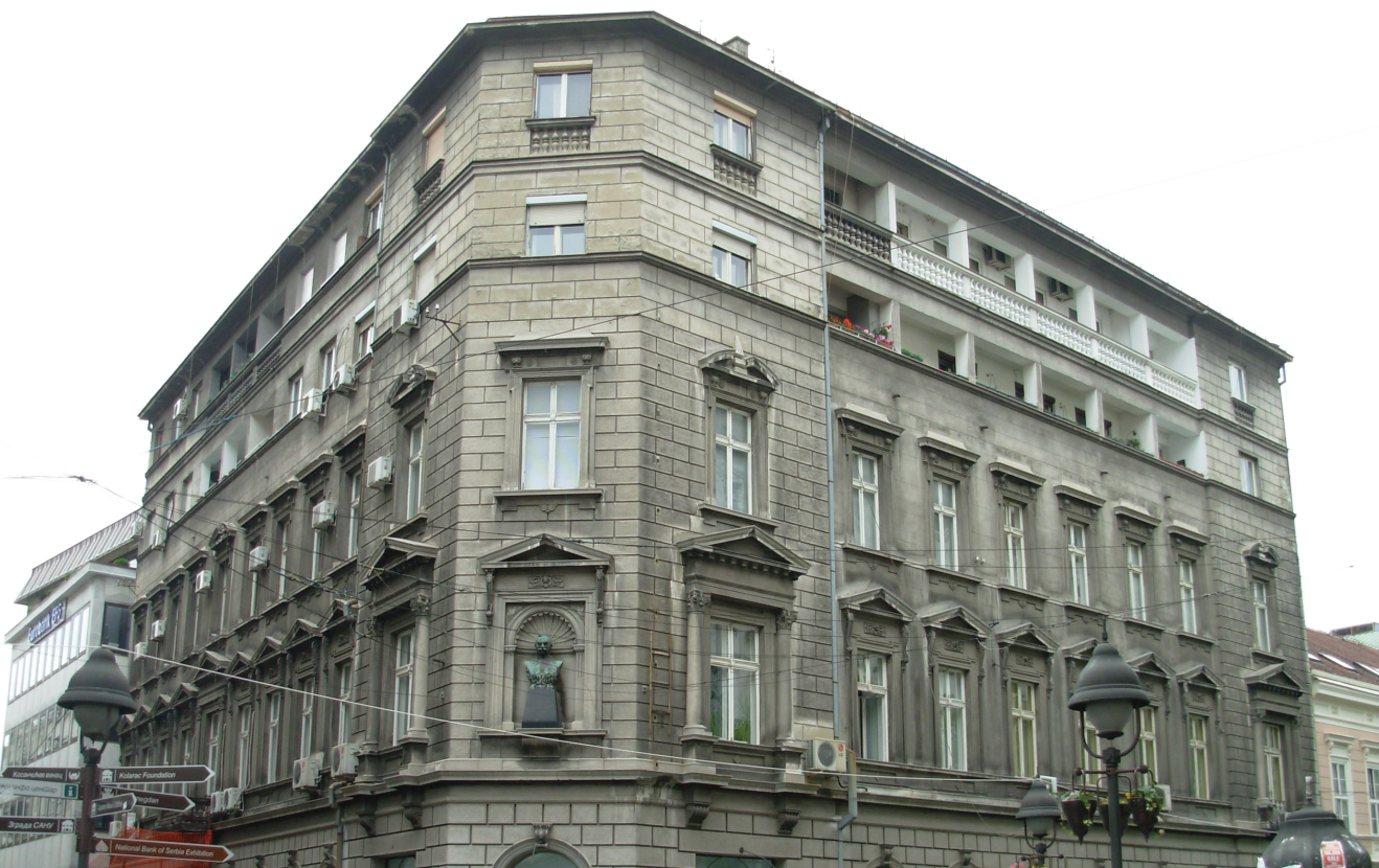
Foundation of Nikola Spasic, Prince Mihailo Street
